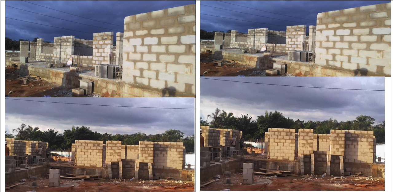
PROGRESS AS AT 30 TH APRIL 2022
